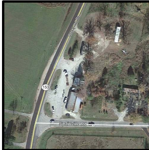
Spainville Store (Landmark #25)
