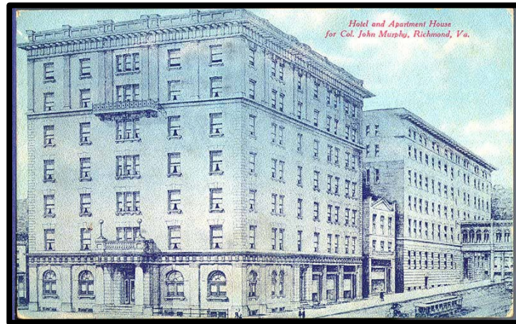
Hotel Murphy at 807 East Broad Street
