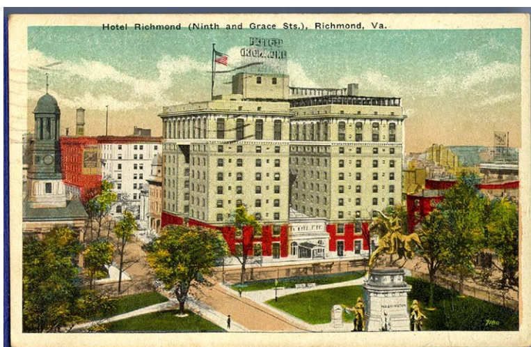
Hotel Richmond After Rebuild
